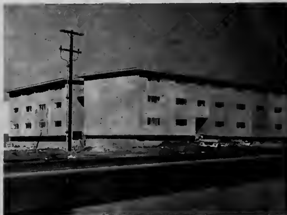
New McAfee Apartments NEAR completion.
